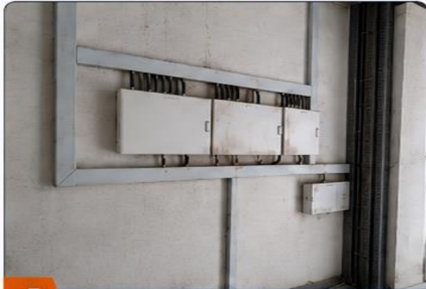
ELECTRICAL DISTRIBUTION PANEL
