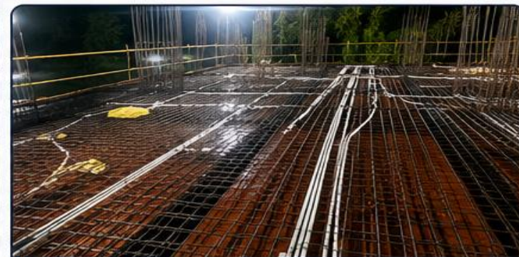
CONDUIT LAYOUT WORK IN PROGRESS
