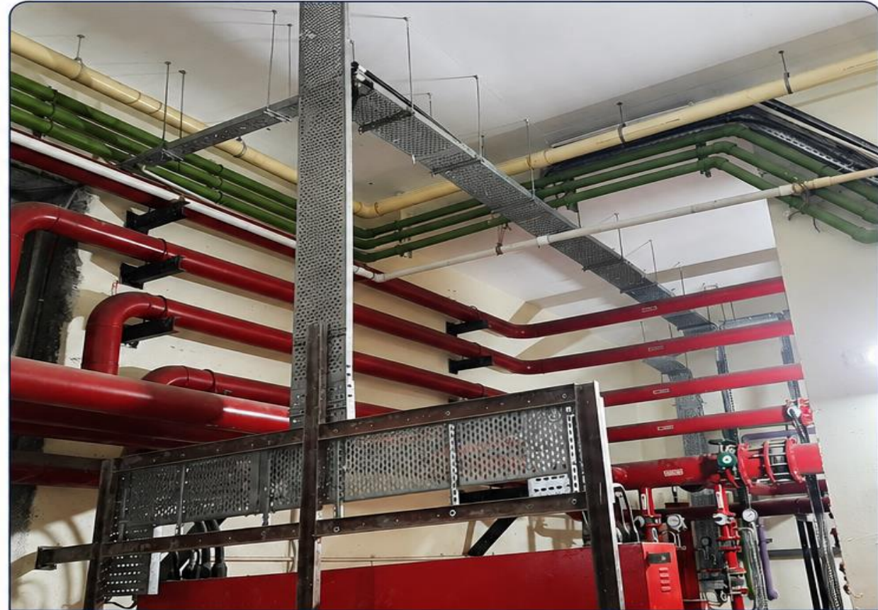
FIRE PIPE & CABLE TRAY INSTALLATION
