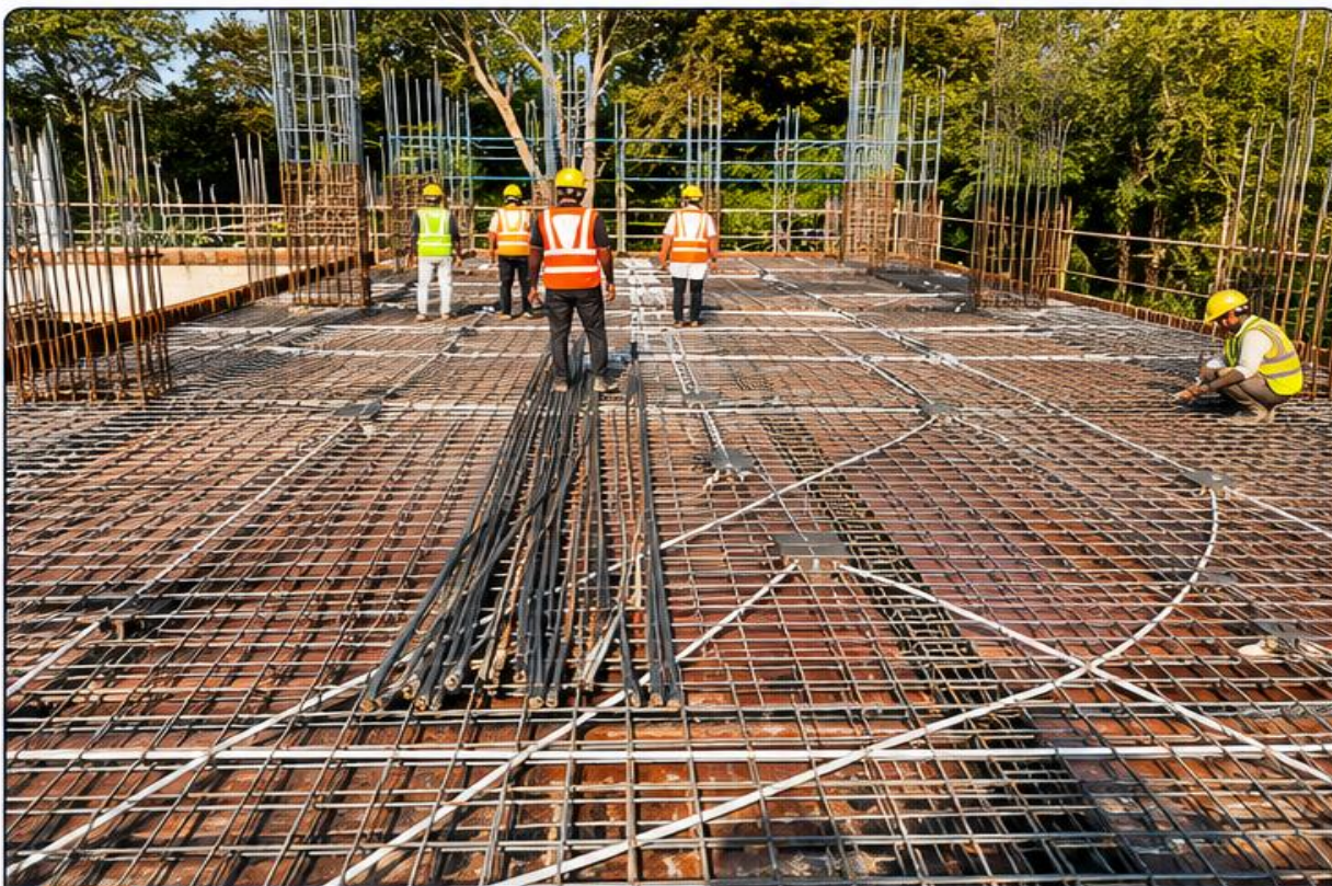
REINFORCEMENT & CONDUIT LAYOUT WORK IN PROGRESS
