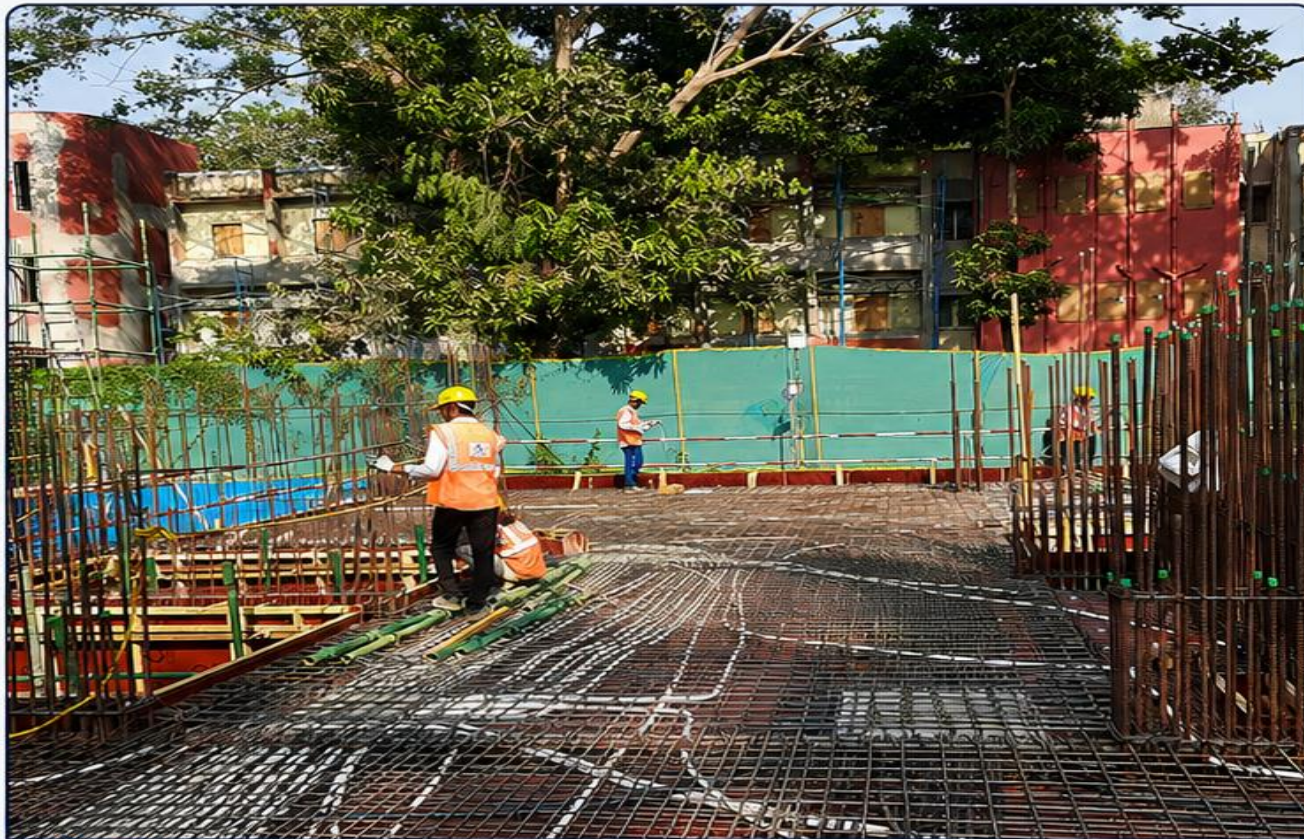
REINFORCEMENT & CONDUIT LAYOUT WORK IN PROGRESS
