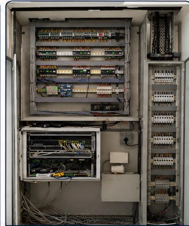
COMMUNICATION & AUTOMATION PANEL
