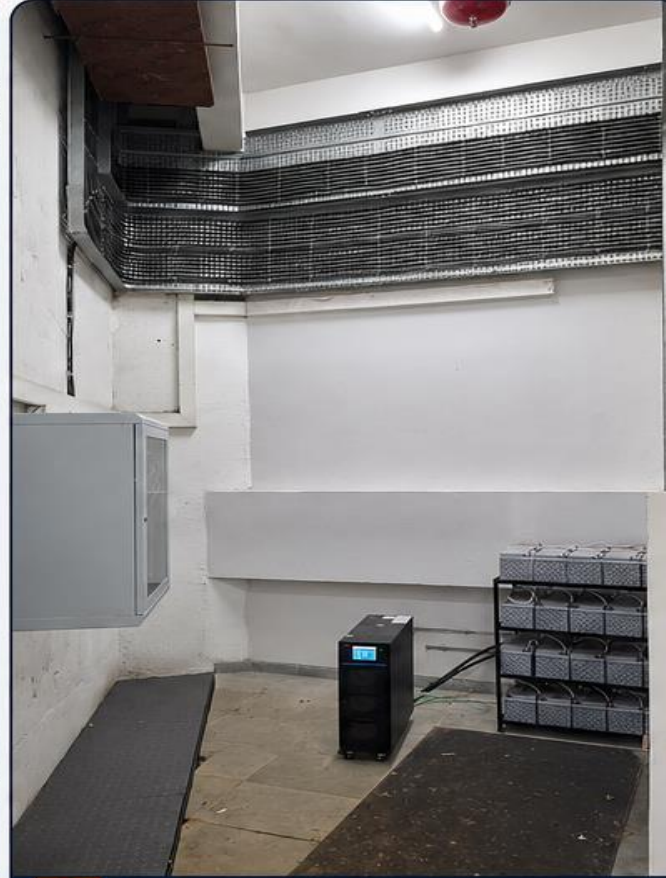
UPS & BATTERY BANK INSTALLATION
