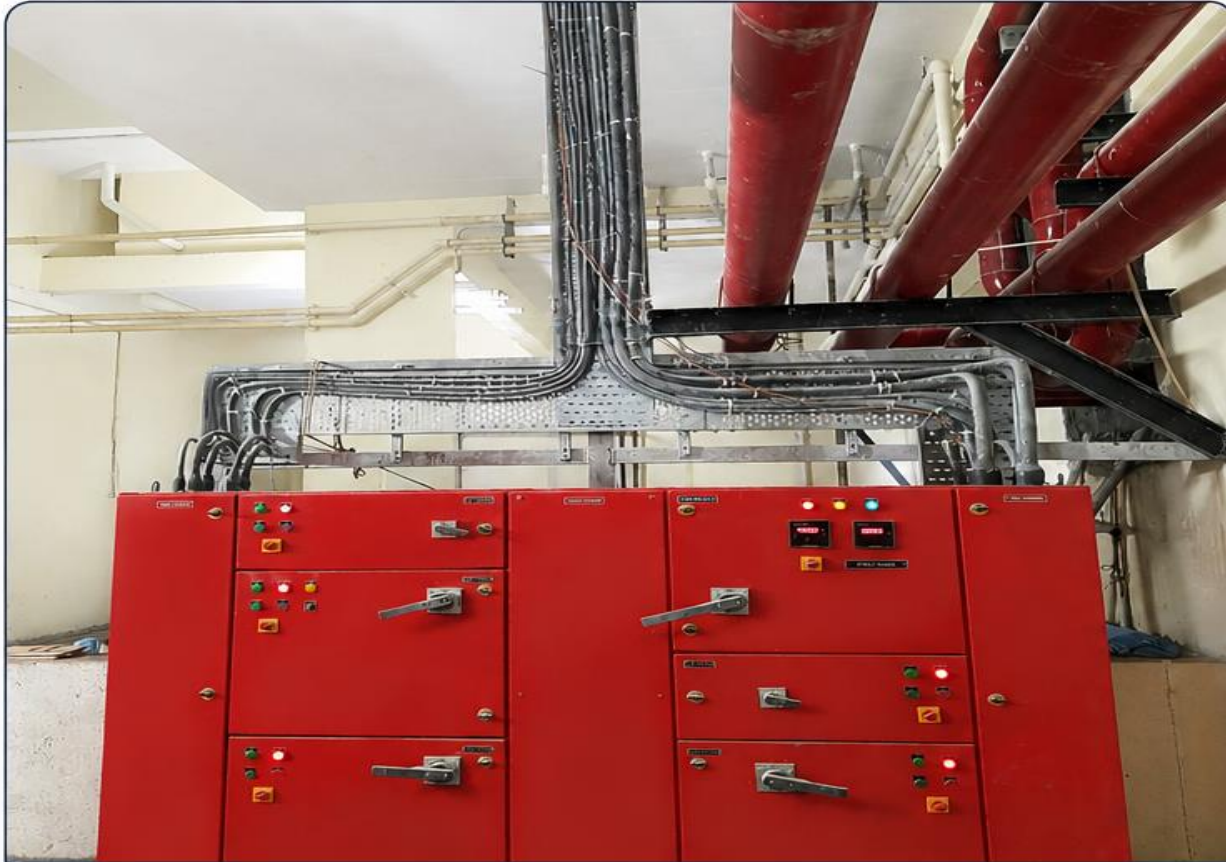
FIRE PANEL & CABLE TERMINATION
