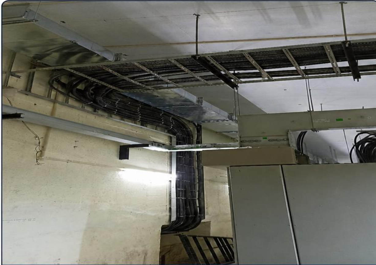
CABLE TRAY & CABLE LAYING
