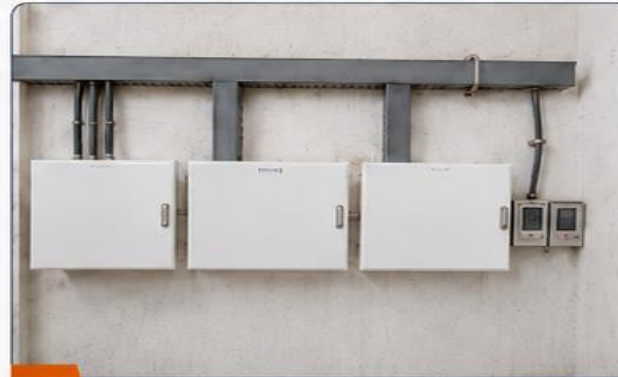
MULTIPLE DB INSTALLATION
