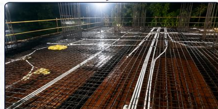
CONDUIT LAYOUT WORK IN PROGRESS
